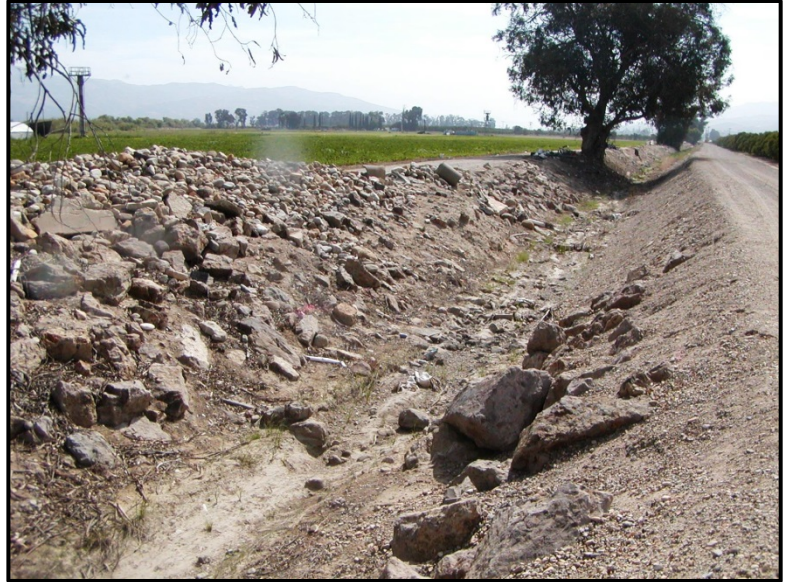
View of site looking upstream
