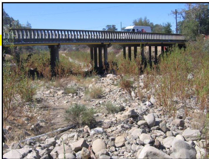
View downstream at the Grand Ave. bridge
