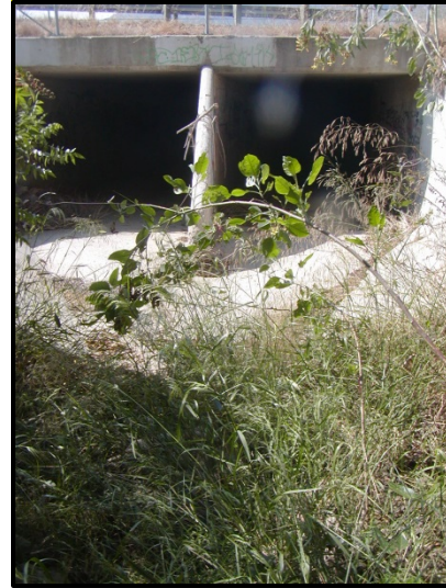
View of site (S) toward Hwy 126
