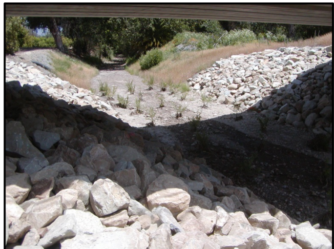
View upstream at the bridge
